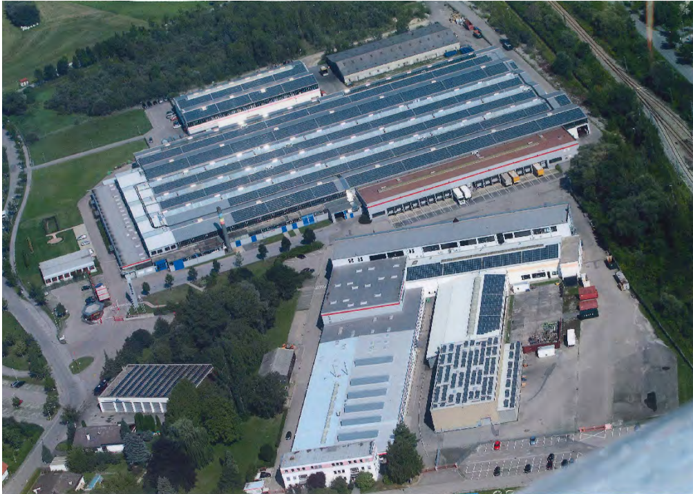
Maximum coverage with PV modules at the Landau an der Isar plant
